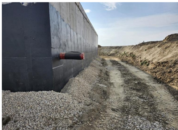
September 12 th 2025: Backfilling around reservoir
